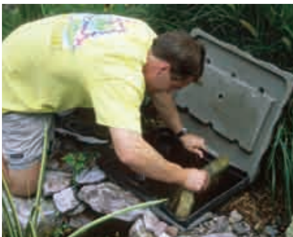
FINDING PUMP PROBLEM: Make sure skimmer net and filter pad are not clogged.
